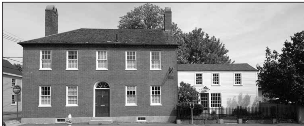
The wooden cottage attached to Jim Reid's in-town residence has been used for many purposes throughout the years.
