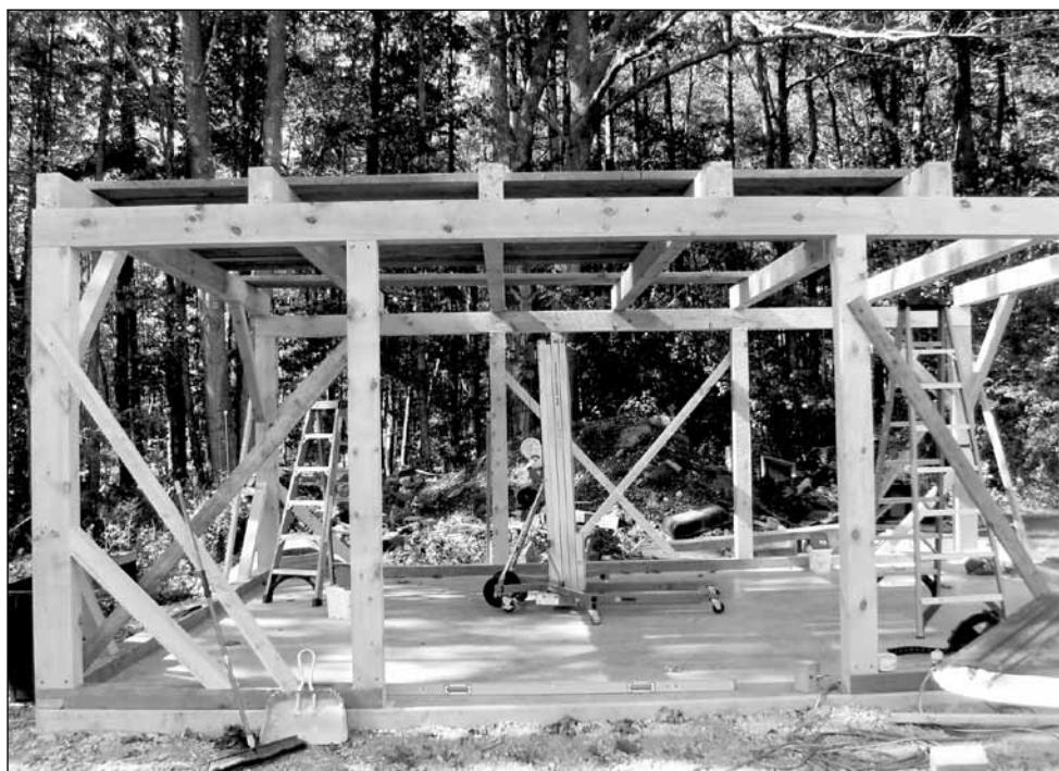
Top: Diagonal bracing is used in the framework to provide support for the entire structure, removing the need for interior load bearing walls.
