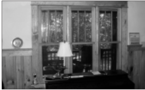
Gregory milled the beads and crafted his own crown moulding for the trim on the Arts and Crafts-style windows.
