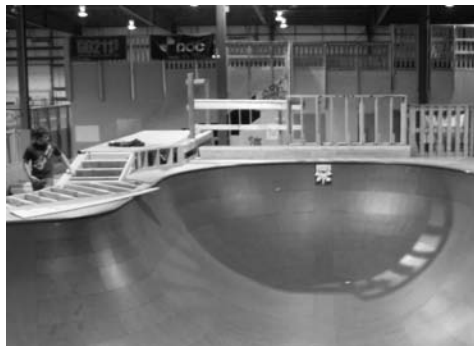
One of the pockets in the park's Clover Bowl was built with two bowed corners..
