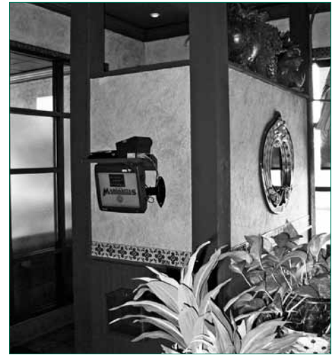
Inside, our one-by-eight rough cut was used to create beams and shelving for wait stations and other partitions.
