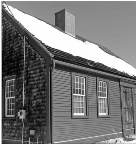
From the shakes on the house's side and roof, to the clapboards on the front, the historic nature of the Pattens' antique cape will be carried through with the new addition.
