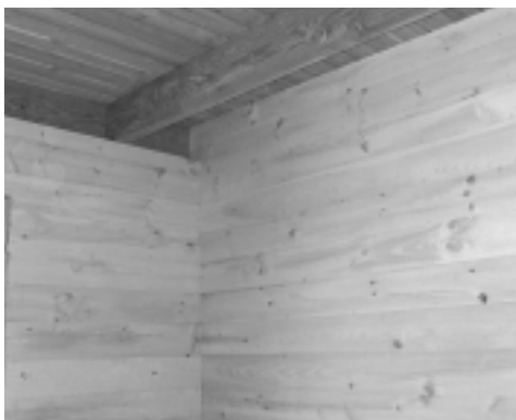
Rand supplied the the rough-hewn pine used in the stalls, custom cut with a band saw.
