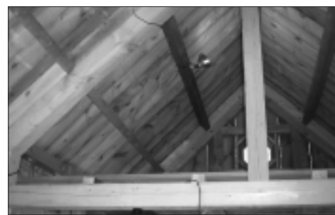
Exterior: Adam Jackson designed his workshop in an antique barn style. Interior right wall: The 16'x24' structure includes rough-cut boards and beams provided by Rand Lumber. Loft: Large 6"x8' timbers provide support as well as a spacious loft area.
