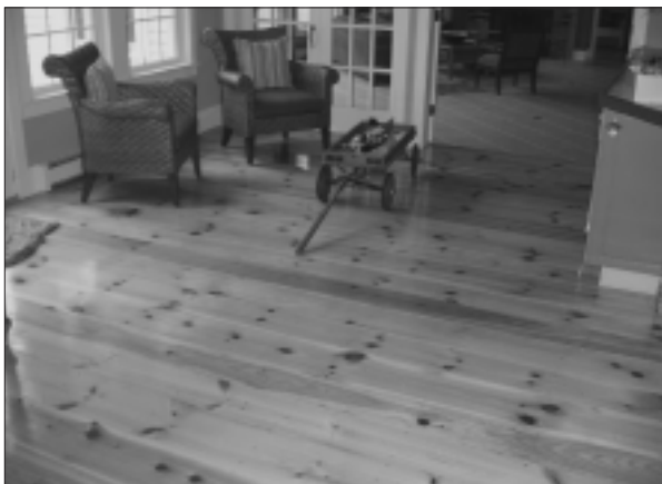
The floor boards were installed with square-faced nails and hand-finished by Steve's mother, Marty.
